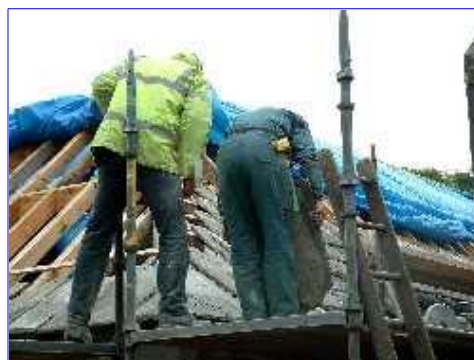
Restoring a steady roof at Pitmuies House
