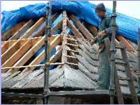
Recycled Carmyllie Flagstone used as a roofing material on steading buildings at Pitmuies House.
