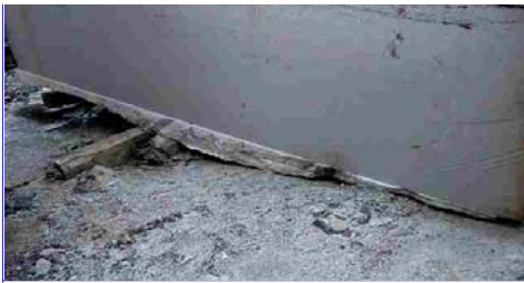
Sample of an early extraction test September 2003
