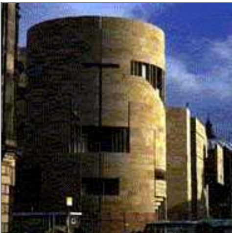
The Museum of Scotland, Edinburgh, designed by Benson and Forsyth Architects.
