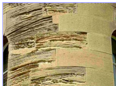
On this replacement stone (Stanton Moor sandstone), the original horizontal bands have been strongly reproduced.
