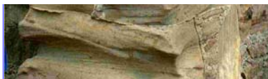
In some areas stone decay is extreme, especially (as here) where the sandstone contains a high proportion of clay minerals
