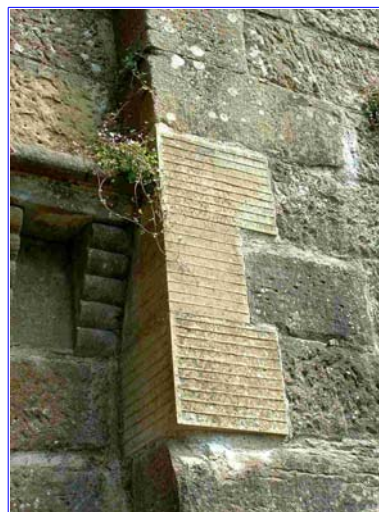
On this replacement stone (Stanton Moor sandstone), the original horizontal bands have been strongly reproduced.
